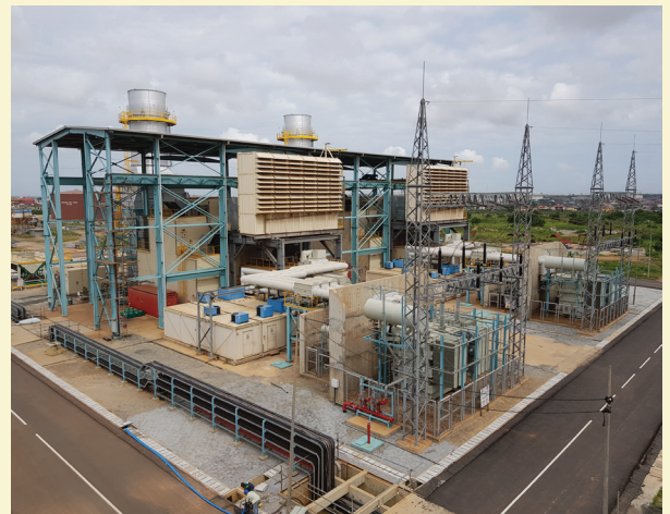
An aerial shot of the gas turbine island.
