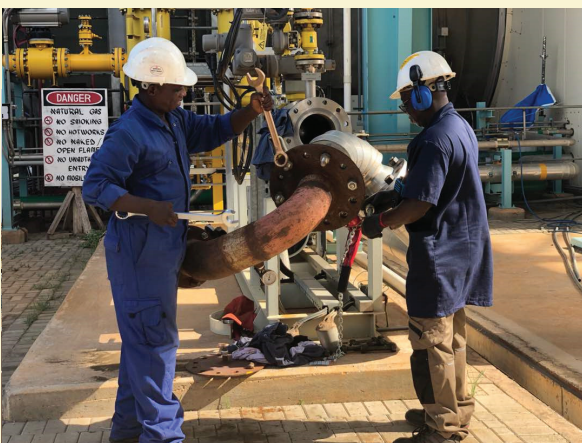
Staff working on the natural gas conditioning facility.
