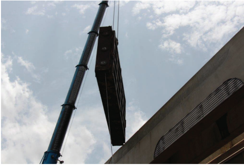
Intake gate being removed from the water.
