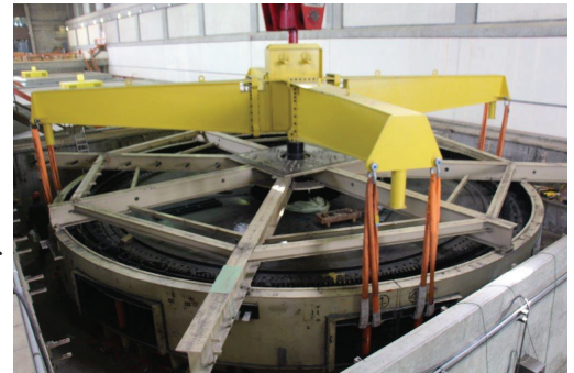
Stator for Unit 3 ready to be lifted.
